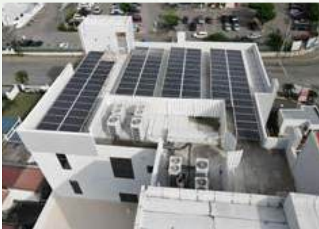
Our most recent 40kw Grid Tie System - 102 Hope Road.
